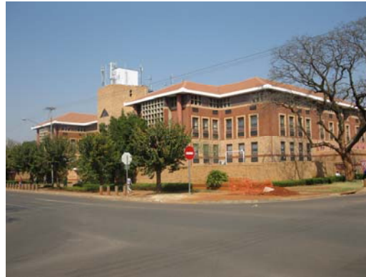
Pretoria Hatfield Sanlam Building
